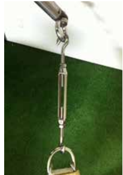
Remove lacing and tension sail into final position
