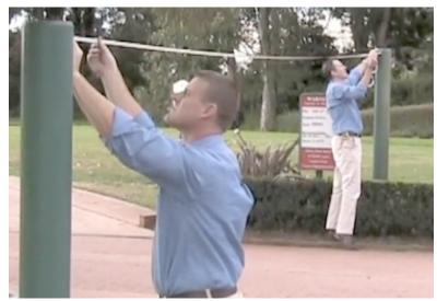
points as point B, C D and so on. For a simple four point rectangular shadesail you simply need to take the point-to-point measurements between each attachment point. Once this is done, you will need to measure the diagonals.
